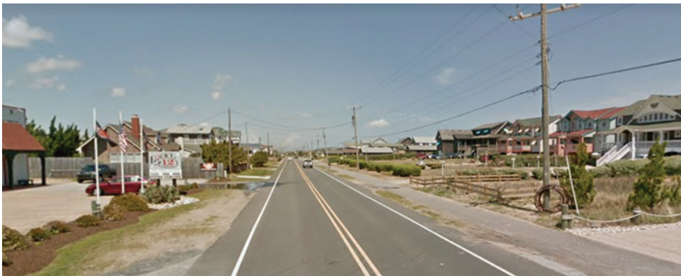
Figure 1 / North Carolina Highway 12, looking northbound
