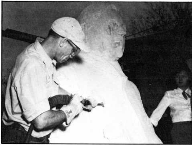
Joe Taylor often had company on the scaffold.
