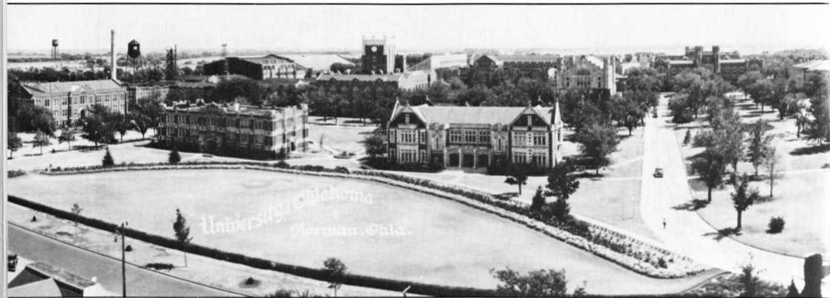
A wide-angle view of Joe Brandt's campus (looking south) shows a University stretching from the Engineering Building on the far left to Holmberg Hall standing just beyond the ivy-covered arches at the Parrington Oval entrance.
