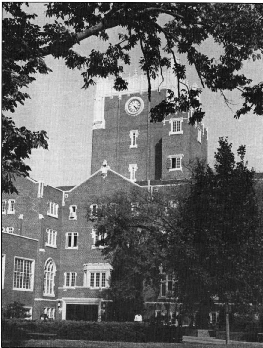
The partially completed Oklahoma Memorial Union was opened in 1929 without the famed clock tower pictured above. A WPA project in 1935 added the landmark to the building, and its carillon bells came as a private gift in 1955.
