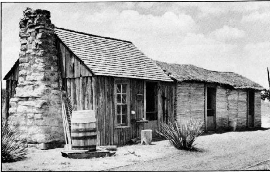
Picket and Sotol House, Crockett County, Texas, circa 1904; relocated to Ranching Heritage Center, Texas Technological University, Lubbock.
