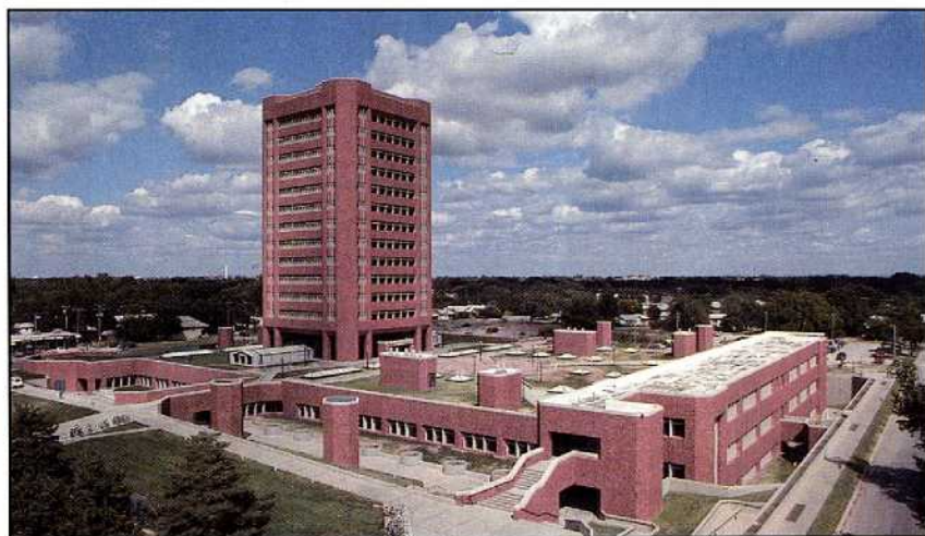
The Energy Center was the project that refused to die. Launched as the oil boom turned to bust, the nine-year construction effort was a tribute to the determination of its backers.
