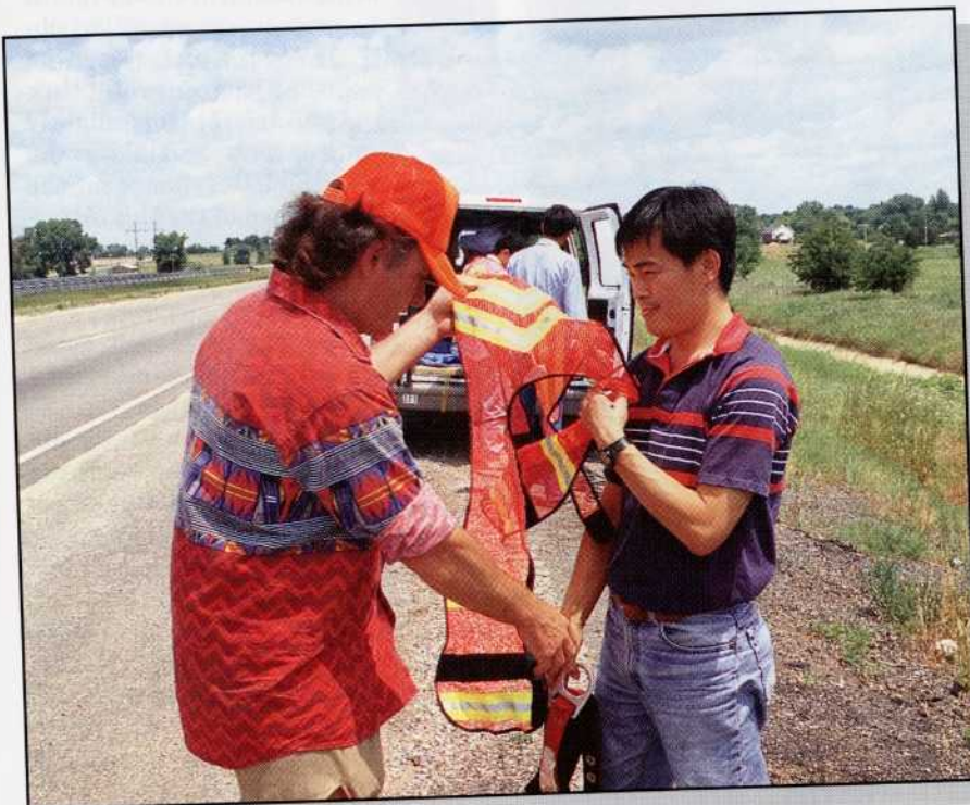
OU engineering professor Bill Patten, left, and C. Mo, a graduate student from Korea, outfit themselves with blaze orange jackets and safety belts recommended by the Department of Transportation for their work at the bridge near Purcell.
