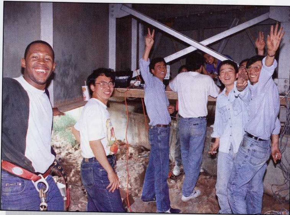
Members of Patten and Sack's bridge team start under the test bridge to check the electronics that have been installed to "shock-proof" the structure.
