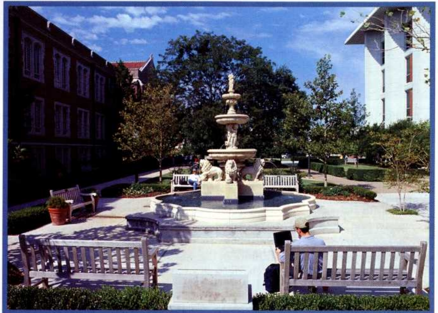
The Fountain Plaza —Centerpiece of Engineers' Court is the Fountain Plaza with this beautiful 14-foot fountain imported from Vicenza, Italy, constructed of a stone local to that area. The court is a series of beautifully landscaped plazas occupying the corridor between Carson Engineering Center and Felgar Hall. The 2,500-square-foot Fountain Plaza was sponsored by James K. and Jerrie Anderson, of Norman.
