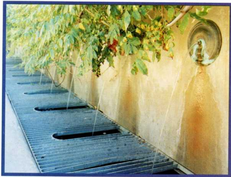
Library Plaza Fountain —Dedication of the E. T. Dunlap Tower and Plaza, with this long wall fountain, occurred in November 1981 before the spring 1982 completion of the adjoining Doris W. Neustadt Wing of Bizzell Memorial Library. The tower and plaza, built with the assistance of the Noble Foundation of Ardmore, honored the longtime chancellor of the Oklahoma State Regents for Higher Education upon his retirement. Also visible from the plaza level is a second small fountain replicating a natural spring in the Canyon Garden, a gift of President and Mrs. Boren, that is located at the bottom of the lightwell area adjacent to the library's lower levels.
