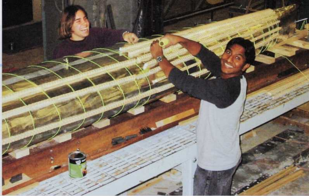
Constructing OU's concrete canoe starts with the mold, here taking shape at the hands of Beth Brueggen, left, and Joseph Thottunkal.
