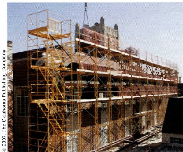
Scaffolding went up on both the east and west sides of Oklahoma Memorial Union this fall to enable construction workers to remove the brick and strengthen support for the horizontal roof beams that were gradually sliding down and pressing against the walls of the building's north extension. Full access to the third-floor facilities closed by the emergency repairs was expected by March.
