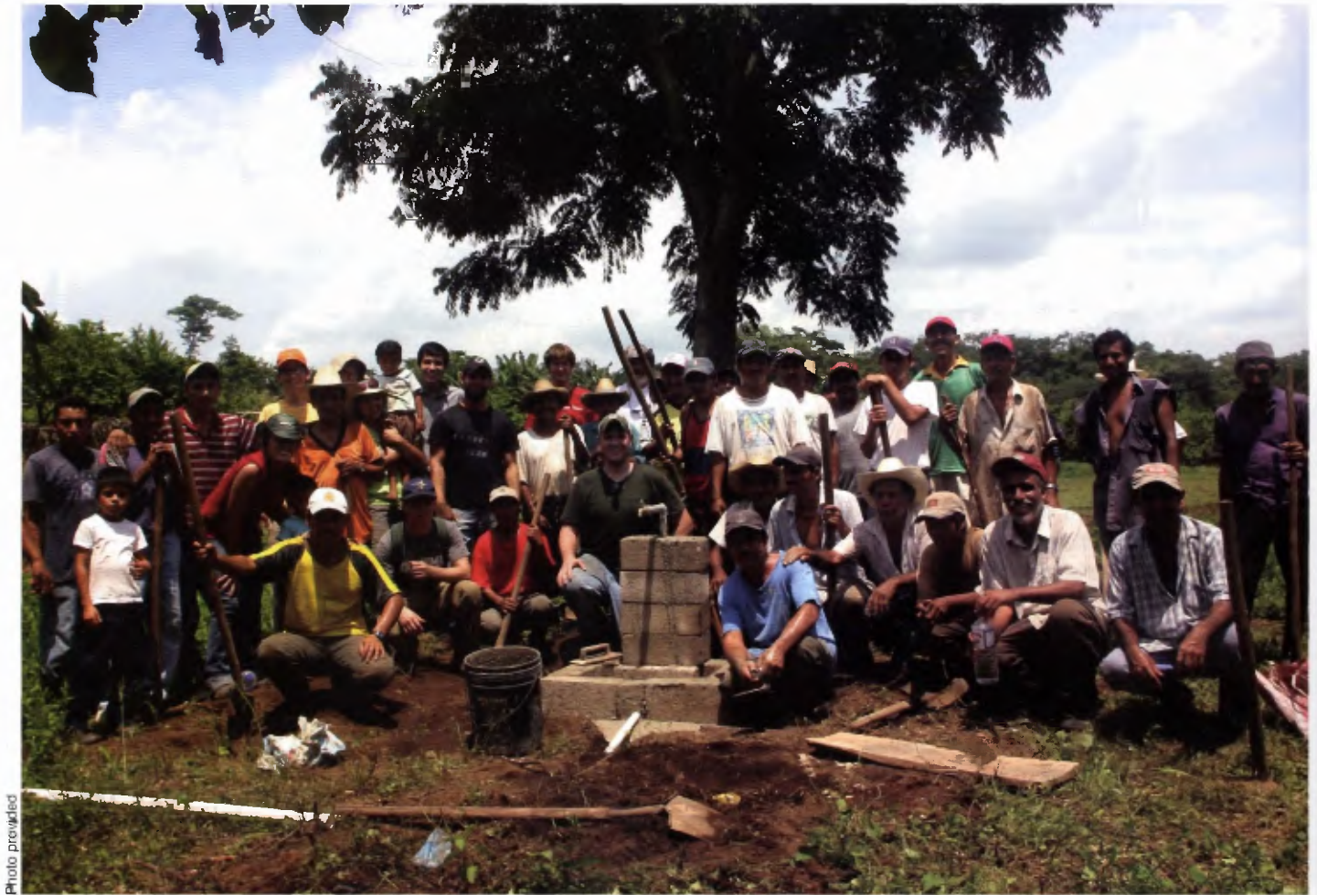
Residents of Pradera del Quetzal, Guatemala, and students from OU's chapter of Engineers Without Borders gather around a completed spring-fed, freshwater pipeline system designed by the students and installed with "sweat equity" from the villagers.
