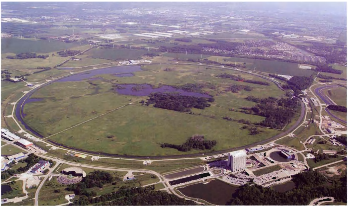
This aerial view of the Fermilab facility near Chicago, a complex consisting of a series of particle accelerators, each feeding the next, shows the Tevatron, Fermilab's highest energy particle accelerator and the location of the DZero experiment involving four OU physicists.
