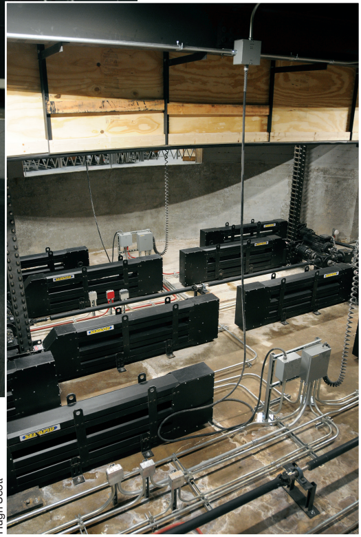
ABOVE RIGHT - The Brackett Theatre’s new Serapid hydraulic system can soundlessly lower the stage lip 17 feet below or lift it an astonishing nine feet above the stage. The lift system was among the most challenging renovation projects, since it was necessary to build an aqueduct to divert a stream that runs below the theatre.
