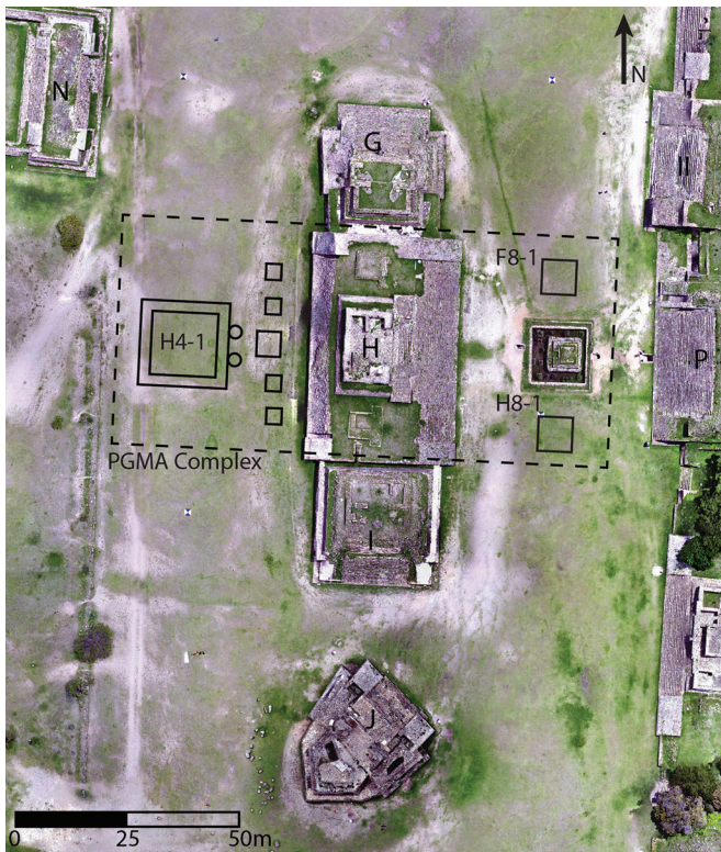
Overhead photo of the Main Plaza, with line drawings indicating the location of buried features discovered—including the remains of what may be a temple.
