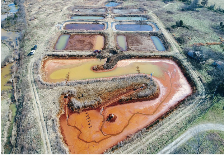
An aerial view from 2018 shows the passive treatment system Nairn and students designed at the Mayer Ranch. The V-shaped pond receives contaminated water from the underground mines. Above, on left and right, are parallel trains of identical treatment units where the scientists can experiment by changing the flow rate, water depth and level of contamination.
