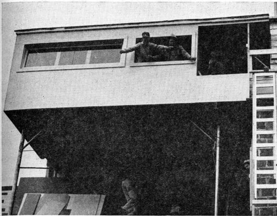
When Bill Stern and the National Broadcasting Company came to the University November 6 to broadcast Oklahoma's 41 to 7 rout of the Missouri Tigers coast-to-coast, a special booth had to be built for Stern, and also for the Columbia Broadcasting System's spot intervals broadcast of the game. Walter Kraft, superintendent of utilities, suggested a porch-like plan which would project the booth out over the crowd in the west stadium without absorbing any of the seats, all of which had been sold since last summer. Here's what NBC's and CBS's temporary quarters looked like while workmen were still in the building process.
