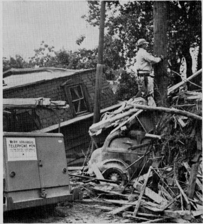
Meeting the Emergency. Telephone people not only worked valiantly to restore service but to keep it going. Dikes were thrown around telephone offices. Switchboards raised above rising waters. Emergency power plants set up. Mobile radio telephones rushed to towns where telephone offices were washed out.
