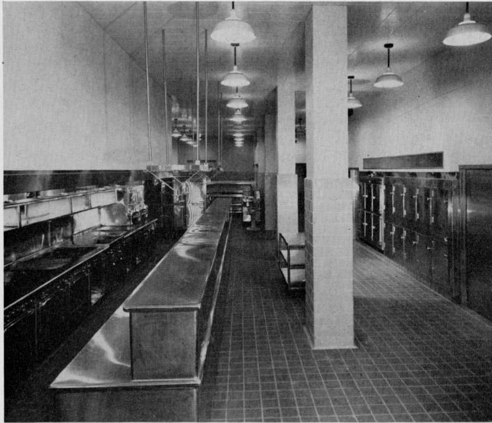
Kitchen of cafeteria is one of the best equipped of its type in U.S. On right are the warming ovens (looks like small refrigerators) for vegetables and bread. Counter in center serves stoves at left. At end of stoves in background are the refrigerators.
