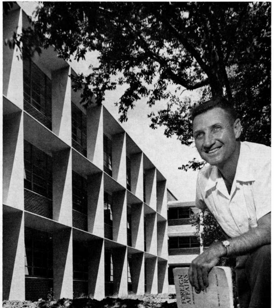
NEW EDUCATION BUILDING, designed to harness sun, wind and light for the benefit of student-teachers, will be occupied for the first time this fall. Dean John R. Rackley, '31ba, '35ma, seems happy with the School of Education's new quarters. Vertical and horizontal triangular shaped baffles of dead-white concrete are the dominating features of the new structure.
