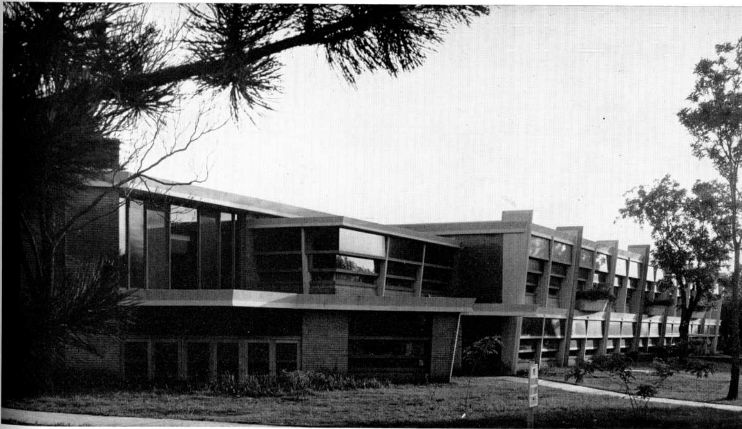
The Home Economics Building was completed in 1951. Constructed of rose brick and glass, structure provides first rate physical facilities.
