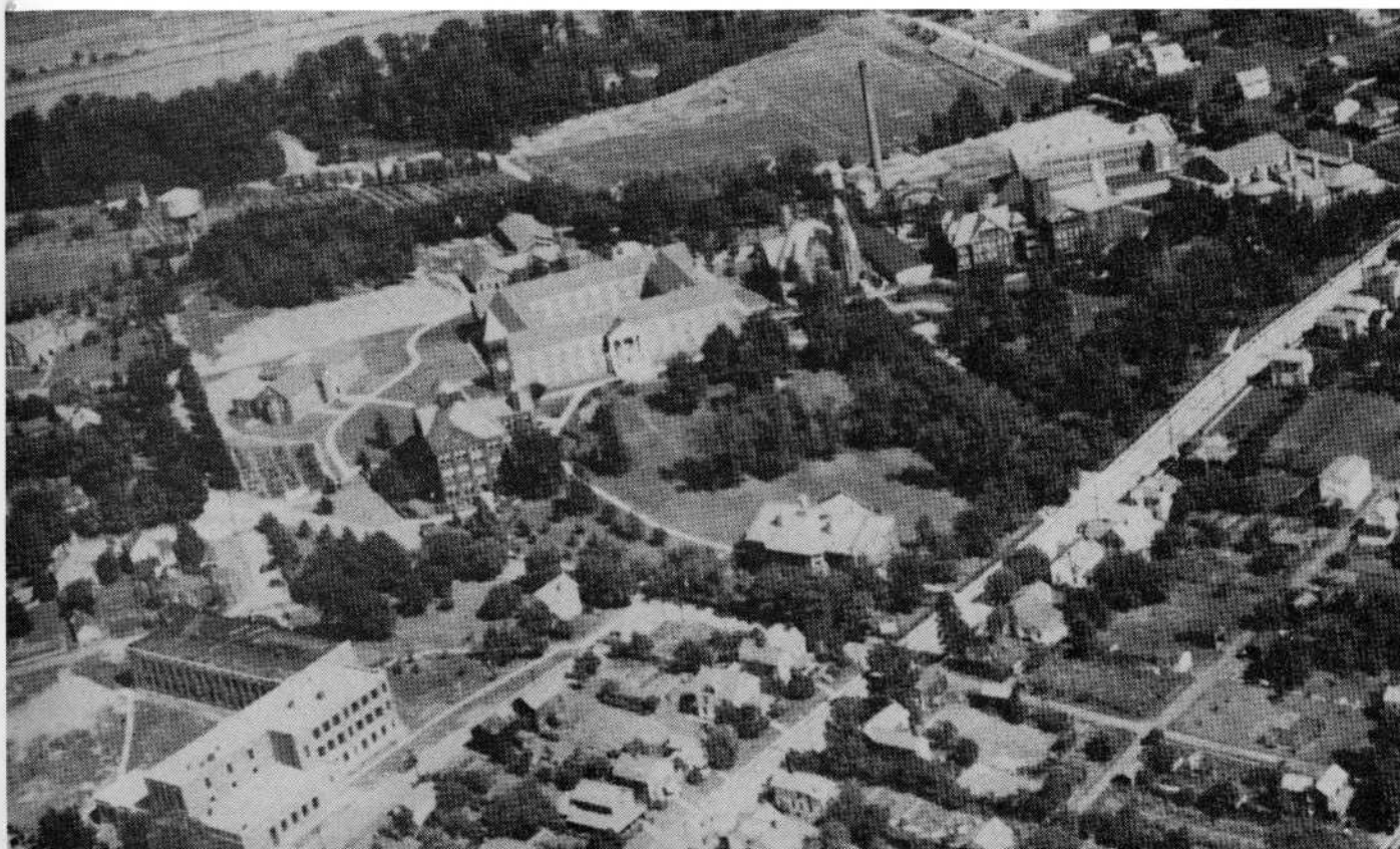
Reproduced from postcard of State Teachers College, Slippy Rock, campus of the small Pennsylvania school shows rolling grounds, major buildings.
