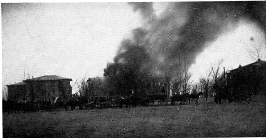
University Hall, the second administration building, burns on December 20, 1907, after a gasoline stove exploded in the dome. Paint being heated on the stove spread the flames.
