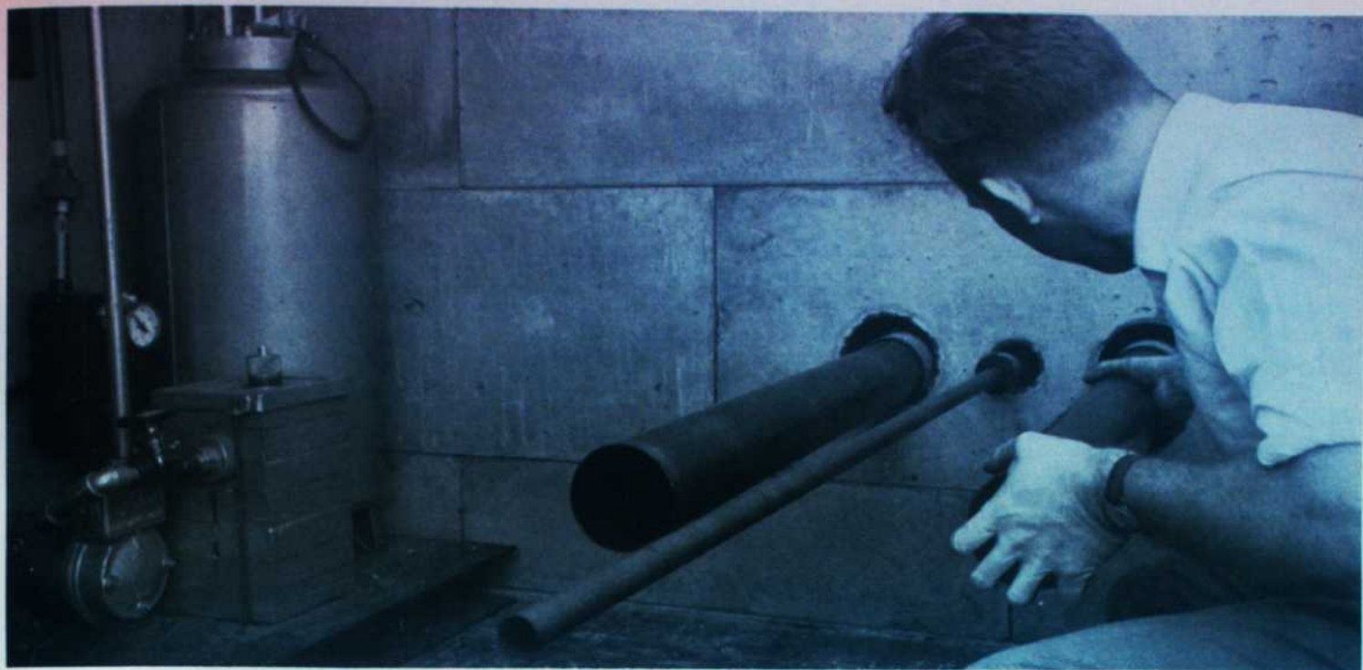
Substances are pushed through these three-inch and one-inch-in-diameter "glory holes" for irradiation in the water-surrounded graphite blocks.
