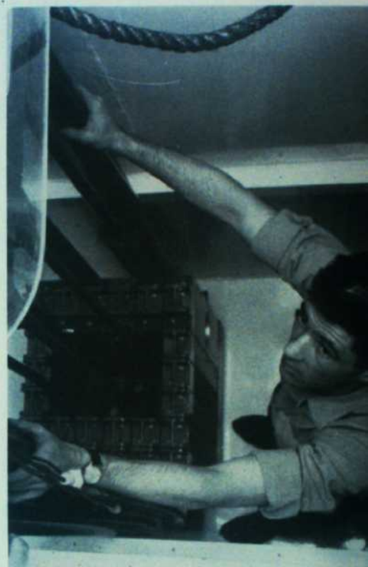
Concrete blocks weighing 1,500 lbs. each are fitted around the reactor's aluminum 'swimming pool.' The tubes are reactor entrances.
