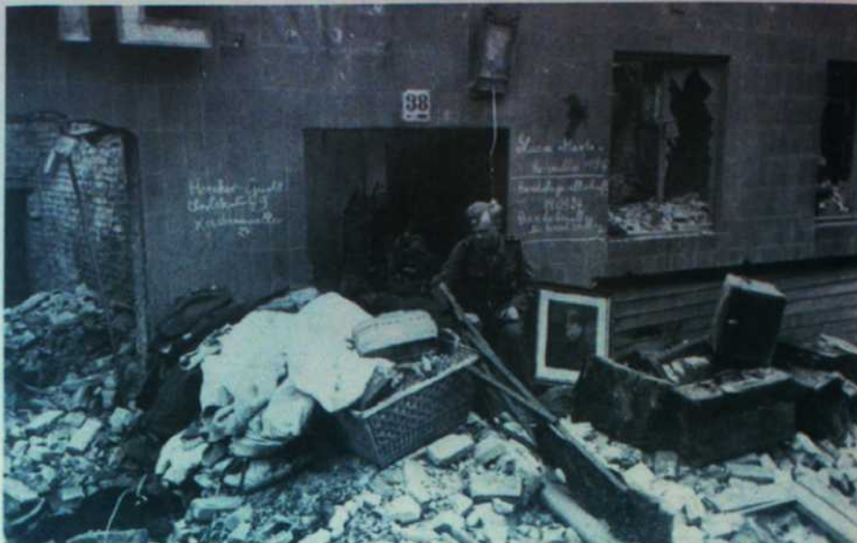
A home's destruction in Berlin. Picture from University Press' Impact of Bomb Destruction .
