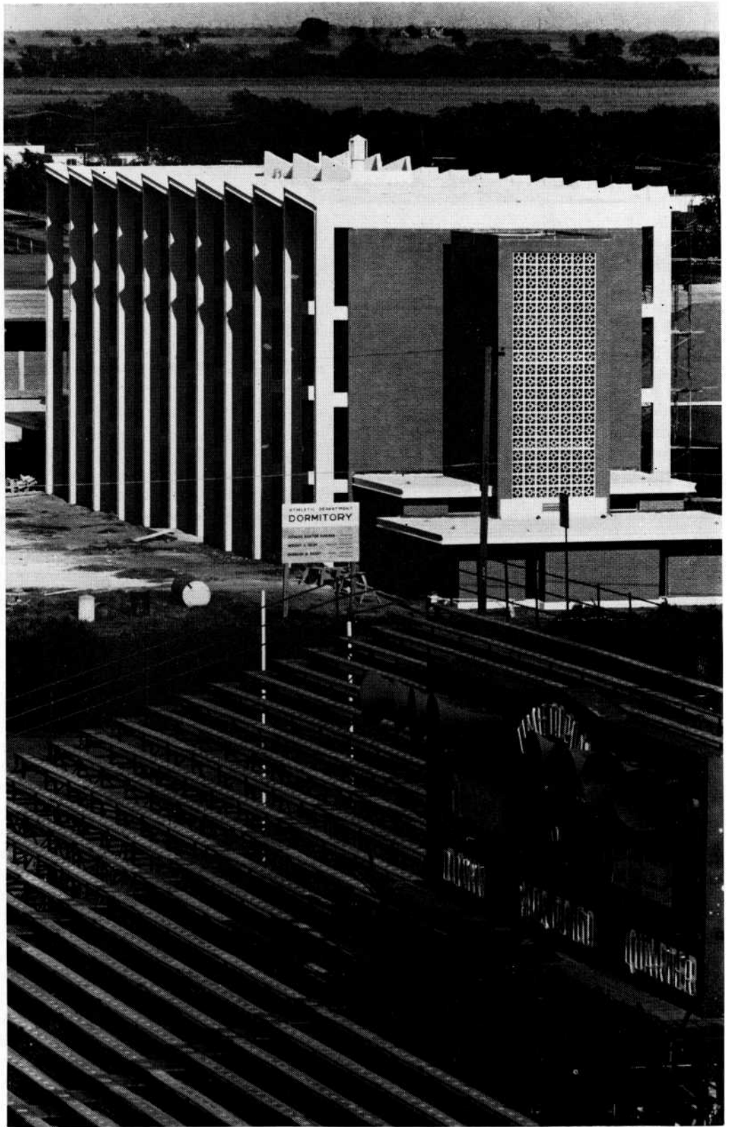
Washington House, new athletic dorm by Barbour & Short Construction Co.
