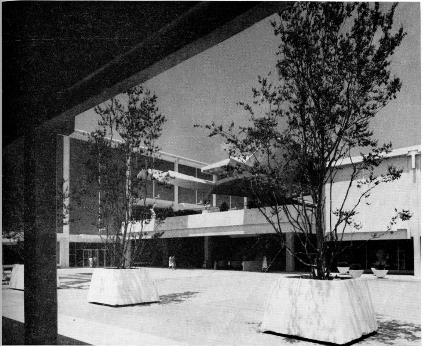
Enough gleaming white concrete went into the construction of Lenox Square to build a 24-foot highway 27½ miles long. By investing in equipment to prepare the concrete on-the-spot and a new "gun" to spray the mixture, Ed Noble was able to cut the cost of concrete construction in half.
