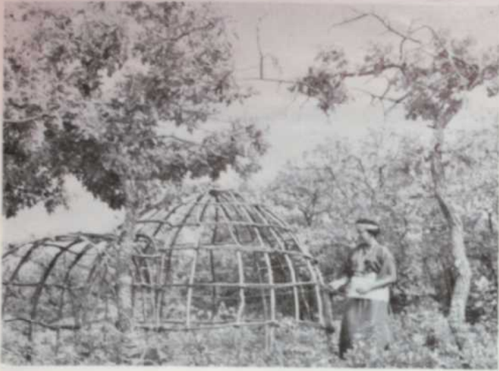
This framework for an Apache wickiup, ready for its covering of yucca leaves or willows, is part of the permanent tribal exhibit.
