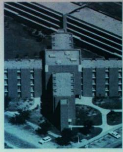
In designing a dormitory, the room comes first, then the grouping of these rooms. Each room in the new Cate Center divides naturally into two areas, while the X-shaped building itself is actually four houses in one. Such construction is more economical and easier to manage yet maintains four identifiable units.
