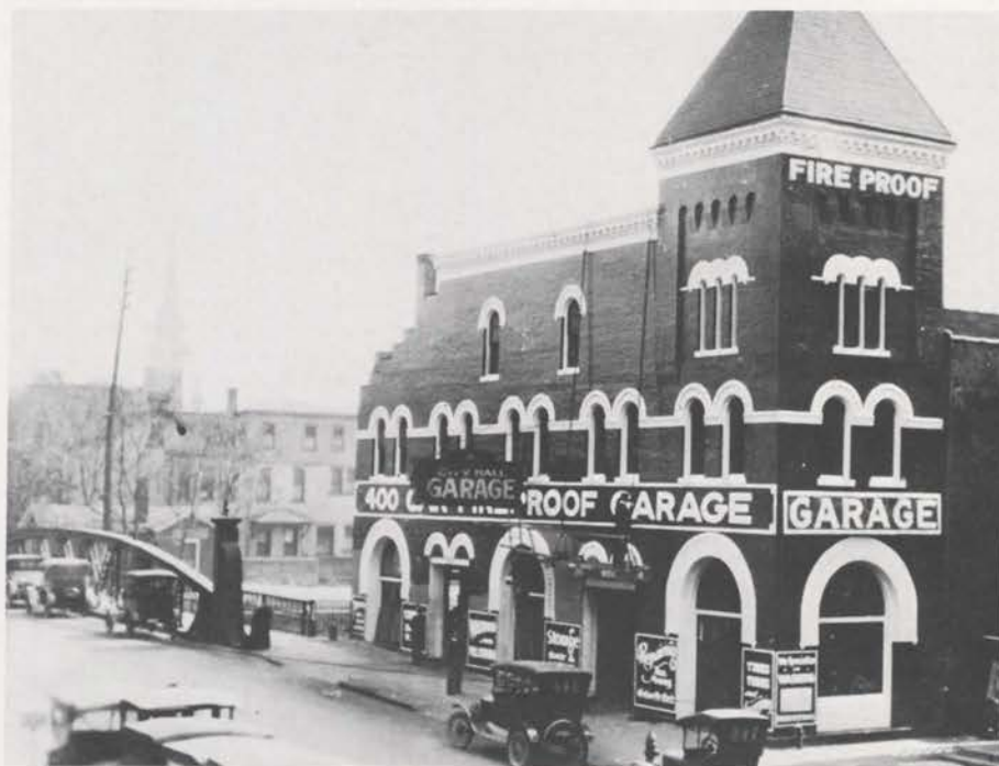
This building once housed Rochester's first Wurlitzer organ. Photo was taken around 1920 when its name was City Hall Garage. Bridge over abandoned Erie Canal bed is at left. Building was drastically cut back when subway and Broad Street were constructed in canal bed. Property is now a parking lot. As far as is known, no picture was ever taken of the organ. —Lloyd E. Klos Collection.
