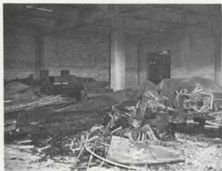
GENERAL VIEW of storage room in which Wurlitzer was placed for safekeeping pending installation.
