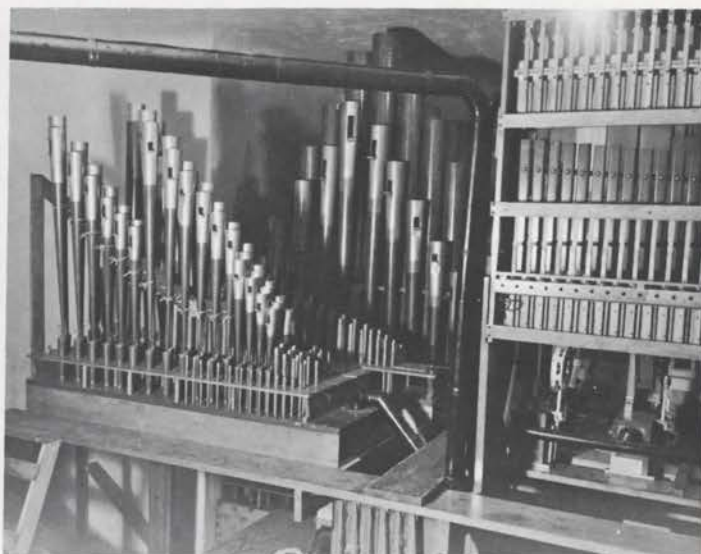
TOP (l to r): Lefthand "Main" Chamber, showing one mitered Violone at left. "Orchestra" Chamber pipework—Oboe Horn, Doppel Flute, Kinura, Saxophone, Solo String, Muted Trumpet. Chamber is in right wall of auditorium. At right, the console drawers at bottom of each jamb house switches to set combination pistons. LEFT: Lefthand "Solo" chamber has a Fern Flute, Viol Ethoria and Vox. BELOW: Left and Right "Main" chamber pipework.
