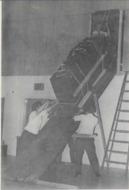
UP THE RAMP! This is how the regulators, switch stacks and relays, tremulants, and chests were hoisted up to the chambers.
