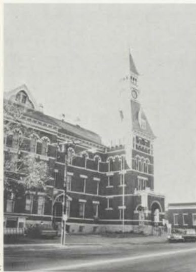
Exterior Thomaston Opera House. ConnValChap organ — 3/10 Marr & Colton installation.
