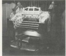
Opus No. 1848, shipped to the Minnesota Theatre in Minneapolis 2/14/28. This is one of two Roman style consoles built, the other going to the Toledo, Ohio, Paramount Theatre. The piano was installed in the Solo Chamber — whereas most were installed outside the shutters. This organ has the single row of stop tablets on the front rail and is now installed in the Reiny Delzer residence in Bismarck, North Dakota.
