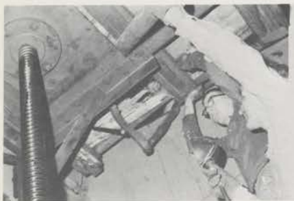
Under the lift.
