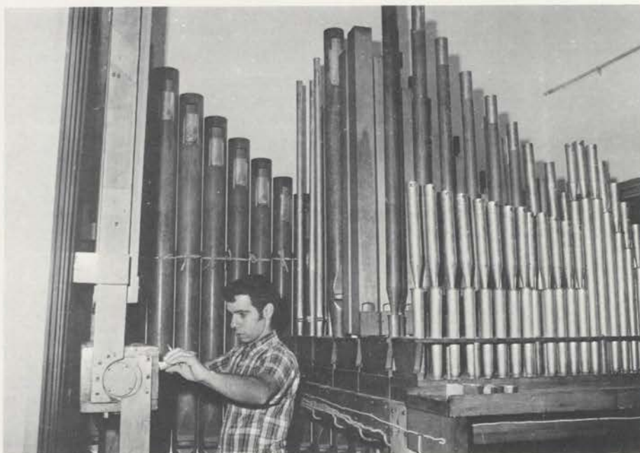
Albert Emola installing wiring on flute chest pipes (front to back): Vox Humana, Clarinet, Open Diapason, Violin, Violin Celeste, 8' Diapason (offset against wall).
