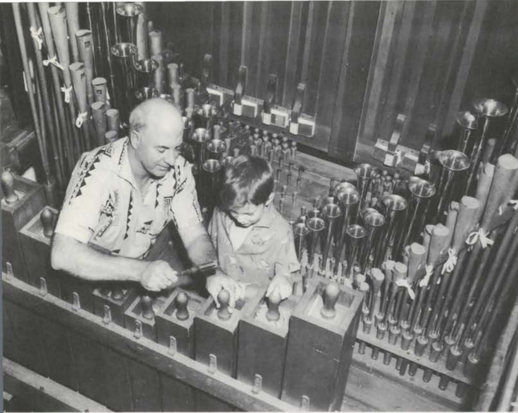
A 1955 photo of Harvey and son Ronnie adjusting a Tibia stopper in the Solo chamber. (W.H. Wilde Photo)
