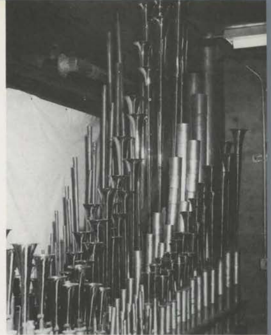
Solo chamber showing from the left: Orchestral Oboe, Brass Trumpet, Quintadena, and Brass Saxophone. Not visible on this chest are the Kinura and Musette.
