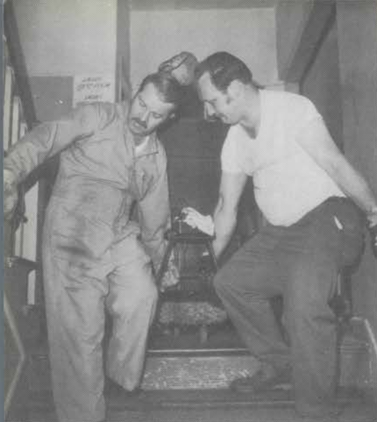
The blower, on a dolly, is edged down a stairway.
