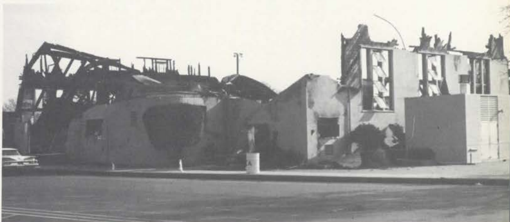
All that remains of the boys' gymnasium. The main school building and auditorium is west of this location. Note the window panes. These are a plastic material which is becoming popular for use in locations where windows are subject to frequent breakage. — (A Carroll F. Harris/Harold Baxter Photo)
