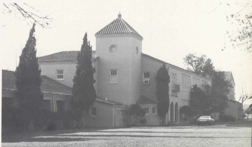
Main building of Grant Union High School. Buildings in this picture are poured concrete external walls with stucco. Arsonists gained entry to the auditorium (extreme right) by breaking a small pane of glass in a front door and releasing the panic bar. Destroyed gymnasium is behind photographer. — (A Carroll F. Harris/Harold Baxter Photo)
