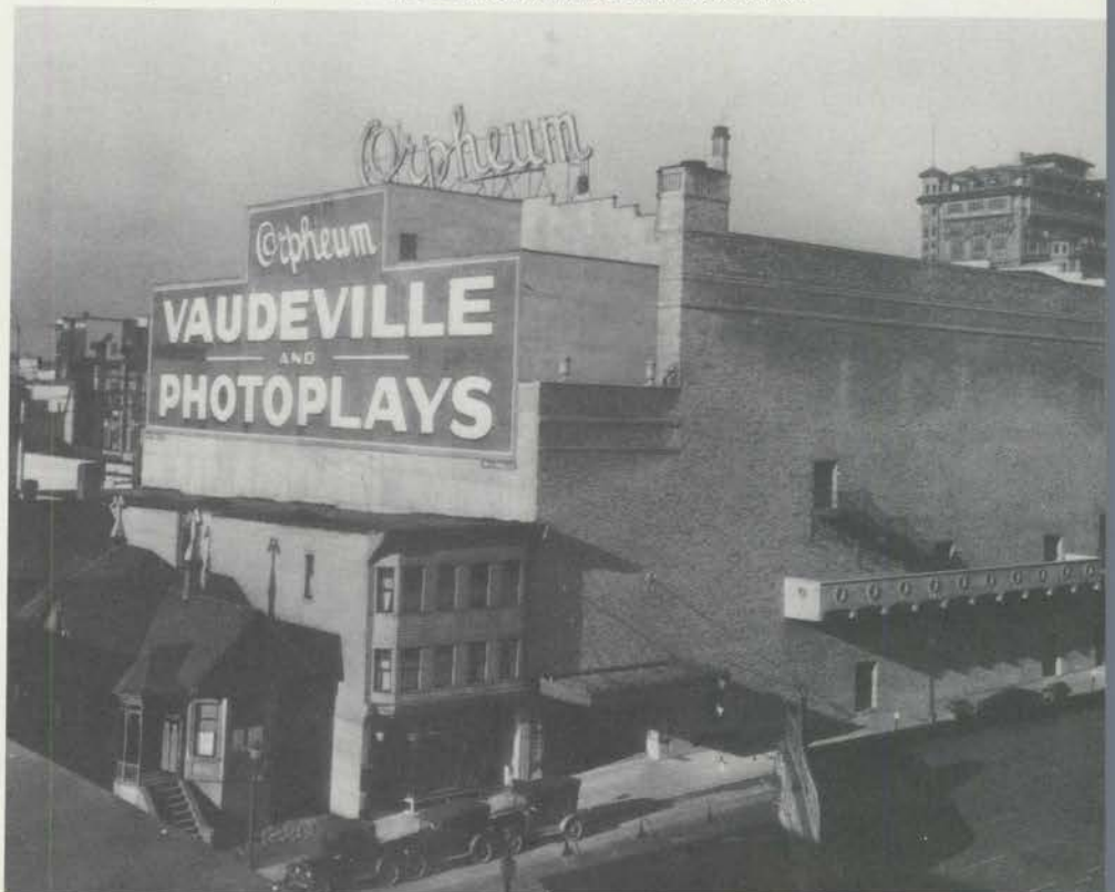
Side view of the Vancouver Orpheum as it appeared at the age of one year (1928). The five story building has actually nine floors, counting from the bottommost cellar.
