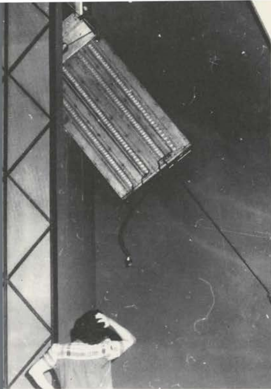
Stand under it and catch it when it comes, Susie! The four-rank chest descends to the church floor, with one-man on the rope, and three more in the chamber guiding it down. An impossible task without Balcom and Vaughn's block and tackle.
