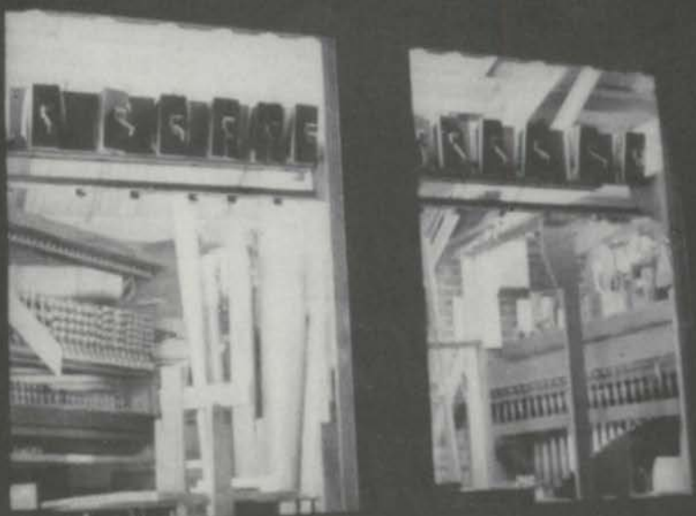
The organ begins to take shape in the solo chamber.
