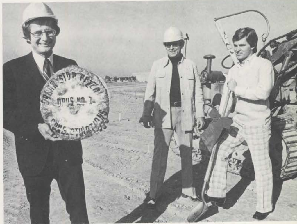
Owner Bill Brown, Tom Rousseau and Ron Rhode at the groundbreaking for Organ Stop No. 2, December 6, 1974.
