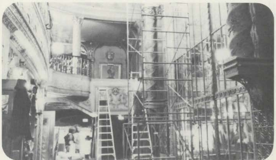
Coronado Theatre lobby during mirror washing day.
