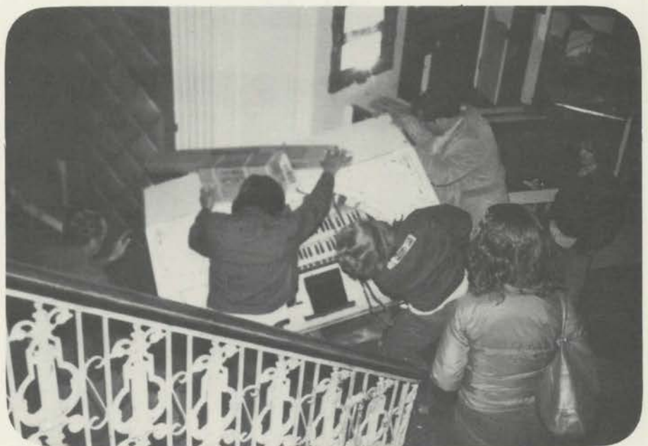
County jail trustees move Capitol Theatre console out through the lobby.
