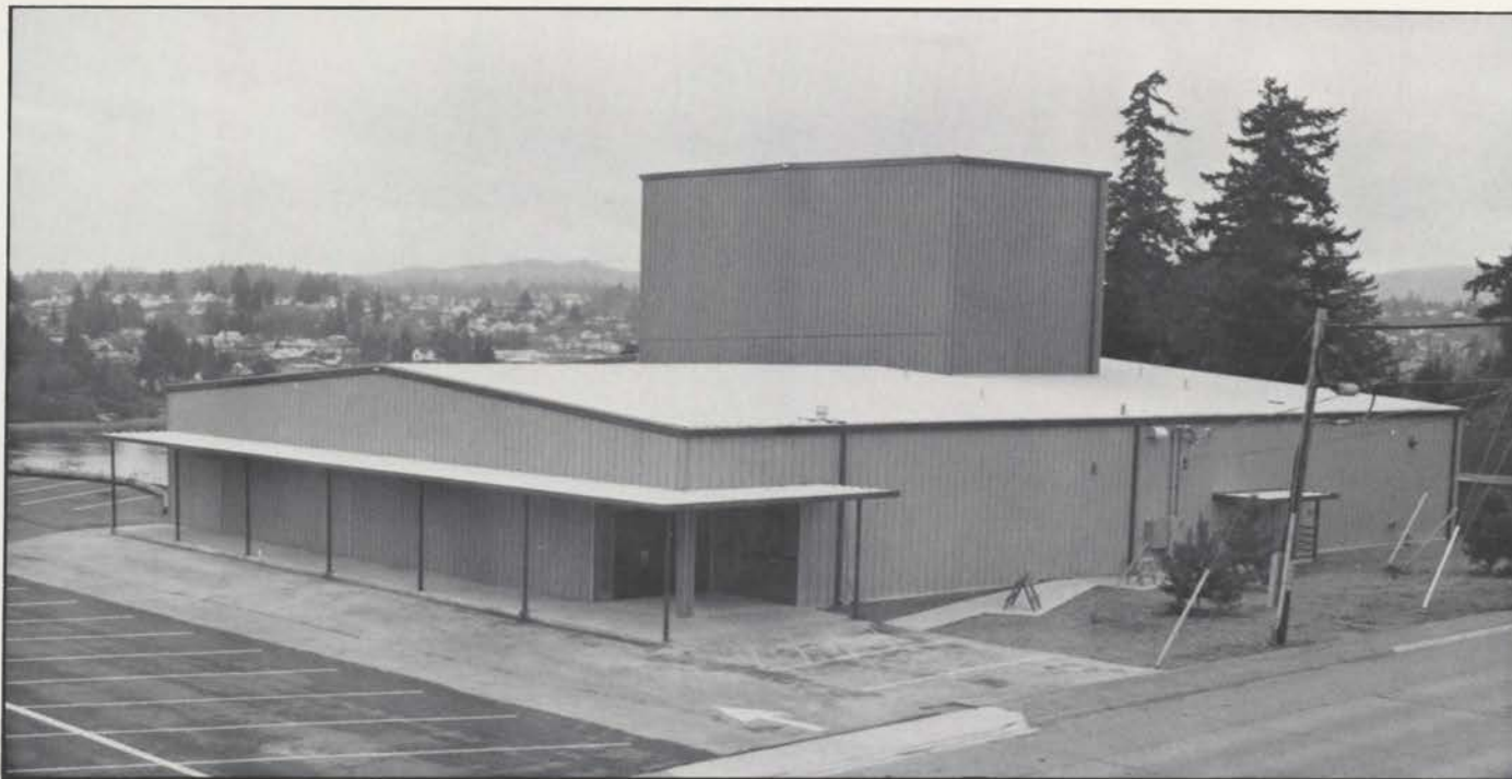
The Community Theatre building was designed primarily as a legitimate stage theatre for the production of plays. Seating capacity is 203. The stage is equipped with a full rigged fly gallery — built mostly from equipment recovered from the Seattle Orpheum Theatre when it was demolished in 1969. Included will be provisions for electronic stage lighting, movie projection equipment, a fully-equipped work shop and scene construction shop, extra rehearsal space and a community meeting place.
