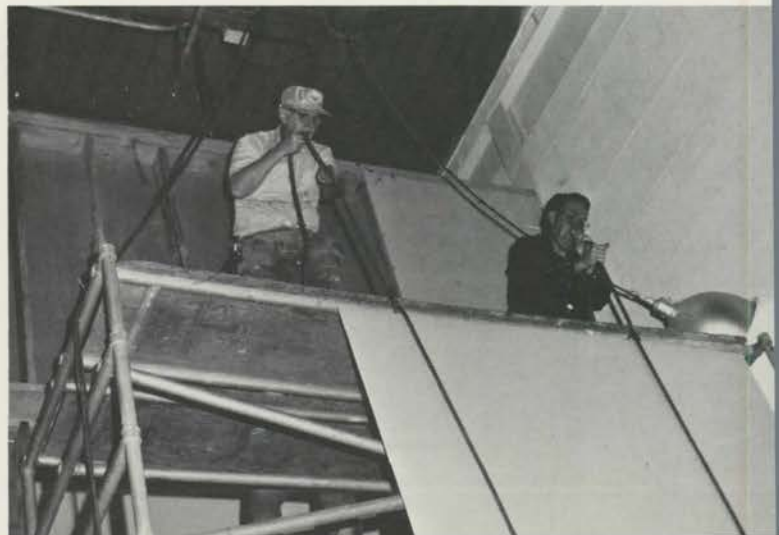
Harold Renico and Ted Decker hoist drywall during chamber construction.
