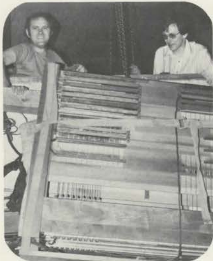
Dave Bishop and Steve McCormick hoist the relay.
