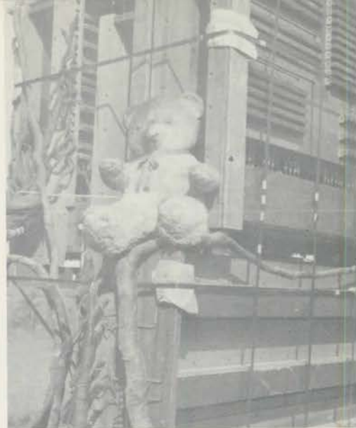
A singed teddy bear guards the switch stacks and relays while they await loading on a truck bound for the Power warehouse for storage. These parts came through the fire almost unscathed because they were located in the cellar — except for water damage.
